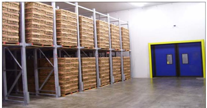
Continuous Duty Ripening Rooms with Galvanized Racking Systems
