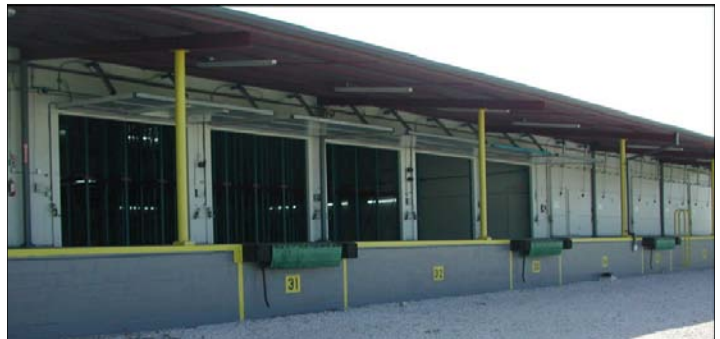
120 Pallet Tomato Ripening Rooms with High Velocity Cooling Units
