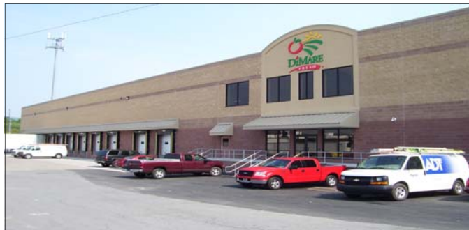
DiMare Fresh, Scranton PA 85,000 SF Distribution Facility
